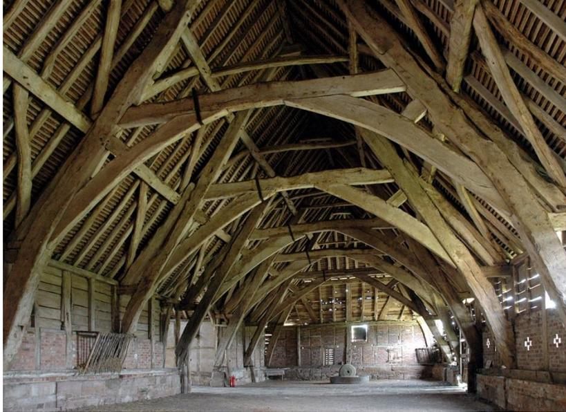
‘Saddles and Skew-pegs: The construction of cruck buildings’
