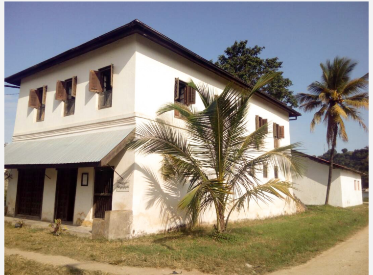
The restored Pangani Heritage Centre, ArchaeoLink
