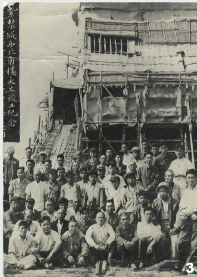
Fig.3 Group photo of the completion of the wooden structure of Northwest Corner Tower Restoration Project in 1957. Courtesy of the Palace Museum, Beijing
